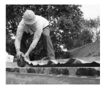
Controlled Expansion Hydrophilic Waterstop for Poured-in-Place and Precast Concrete
